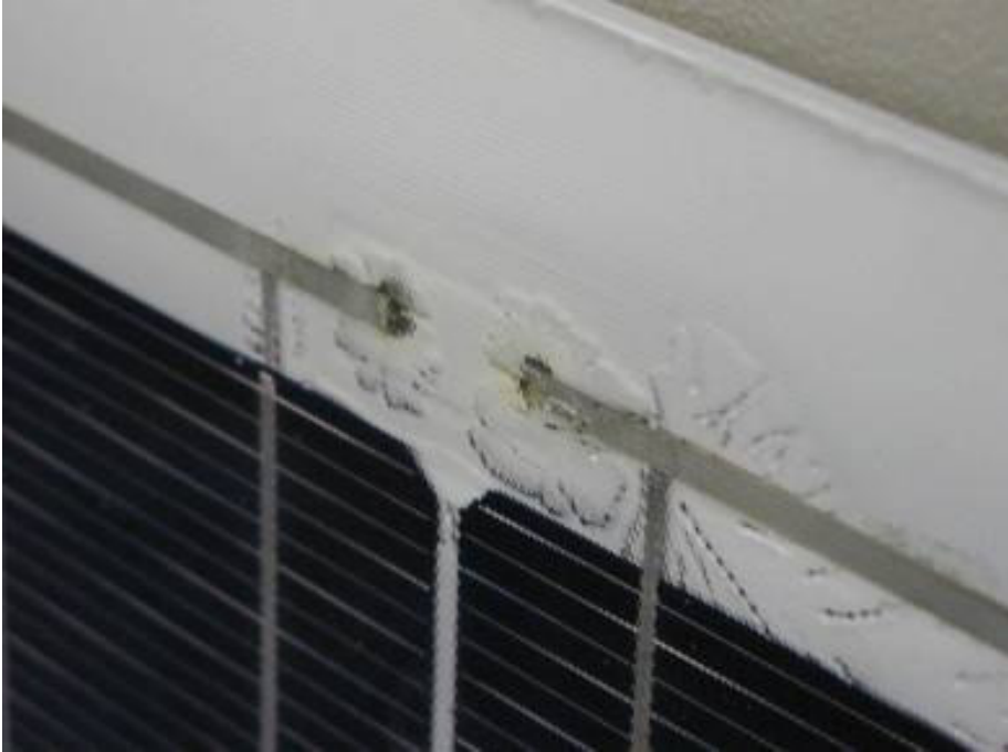
Insufficient lamination quality
